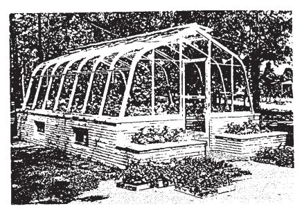
A free-standing greenhouse is set apart from other buildings, with a door at one end (or a door in both ends for long units).
